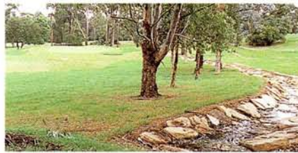
Sealed rock lined channel to divert flows around the fairway.
