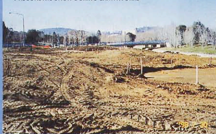
PRECONSTRUCTION DURING EARTHWORKS
